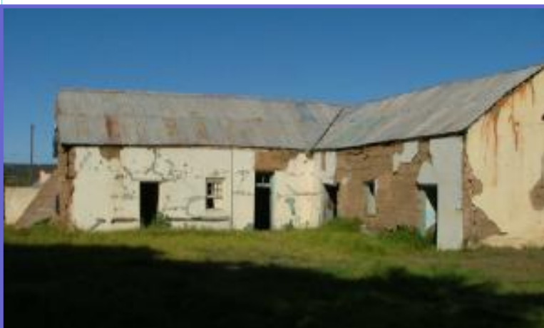
2004: A seriously dilapidated Opstal in need of considerable renovations
